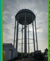
Notice a difference in the skyline in your neighborhood? Our Bethel St. water tower is getting a makeover! The brackets as shown are tarp containment brackets. When it's time, a tarp will be placed over the water tower to mitigate debris from sandblasting and paint overspray on neighboring properties and these brackets will help hold the tarp in place. Follow our Facebook page for more updates on the progress of the water tower makeover and to see the final product!
